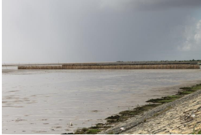
Figure 16: Completed Walton Hall Brushwood Dam sediment trap
