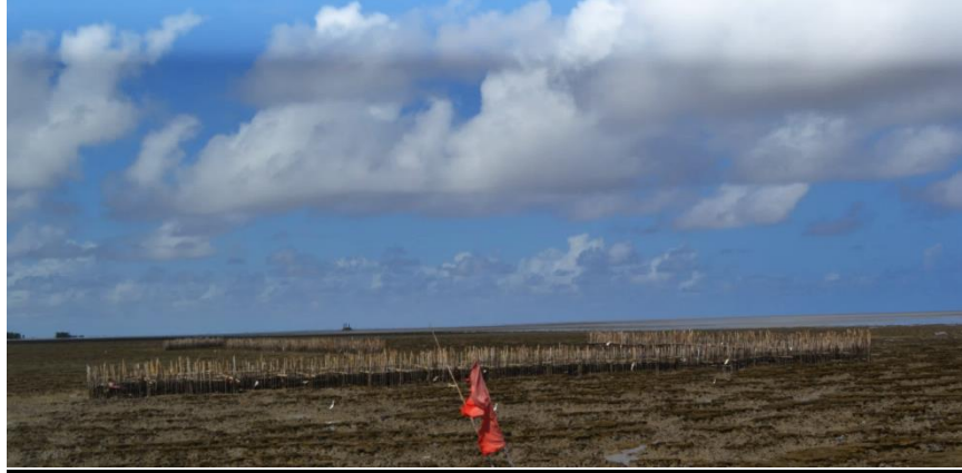
Figure 18: Completed Lusignan brushwood dam
