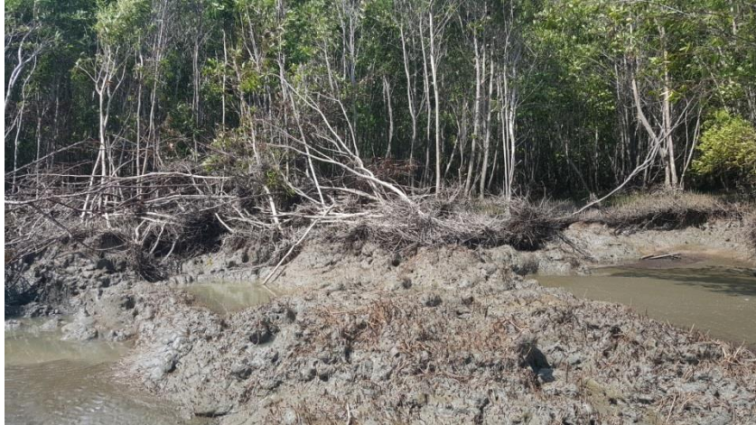
Figure 7: Erosion at Hope Beach, ECD
