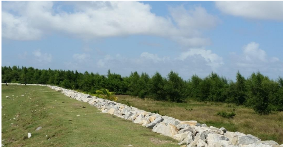
Figure 3: Devonshire Castle, Essequibo Coast, Region #2, Geotextile tube groyne
