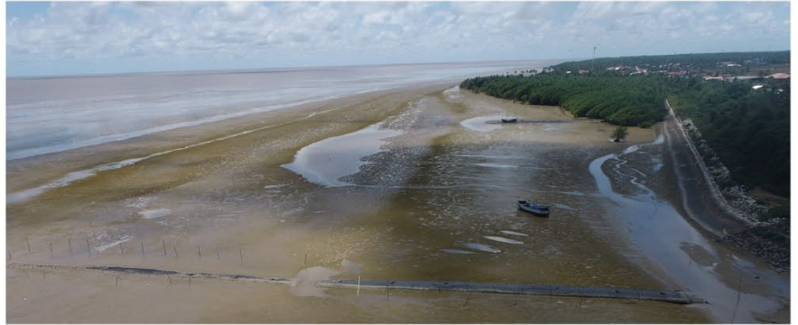
400 meters geotextile tube groynes completed at Exmount, Essequibo Coast, region 2
